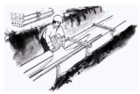
6. GILSULATE® 500xR is a light colored dry granular material. To minimize dust, empty bags on pipes with as little "free fall" as possible. Fill trench to mid pipe height and consolidate. Remove spacers and temporary pipe supports as work progresses. Coat anchors, guides, supports, wall entries with bitumastic as specified just prior to placement of GILSULATE® 500xR.
