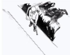
7. Add additional layers of GILSULATE® 500xR and consolidate to specified thickness and density. A rod-type concrete vibrator with a 1<sup>1</sup>/2" or smaller diameter head is the best and quickest means of consolidating GILSULATE® 500xR. Insert the head of the vibrator horizontally and pull along slowly. Larger pipes require consolidation in two or more lifts of material.
