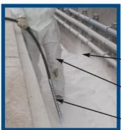
NARROW TRENCH REDUCES EXCAVATION. 24" CWSR, OUTSIDE CFUD THICKNESSES 6" PIPE SPACING 6"
